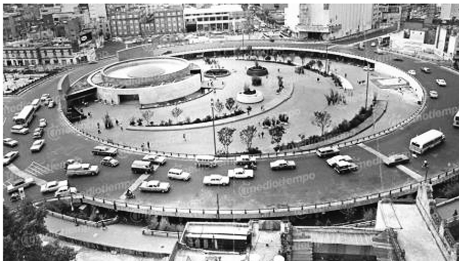
Fig. 2. Insurgentes metro station 1969. This station was a location in the futuristic movie Total Recall.
